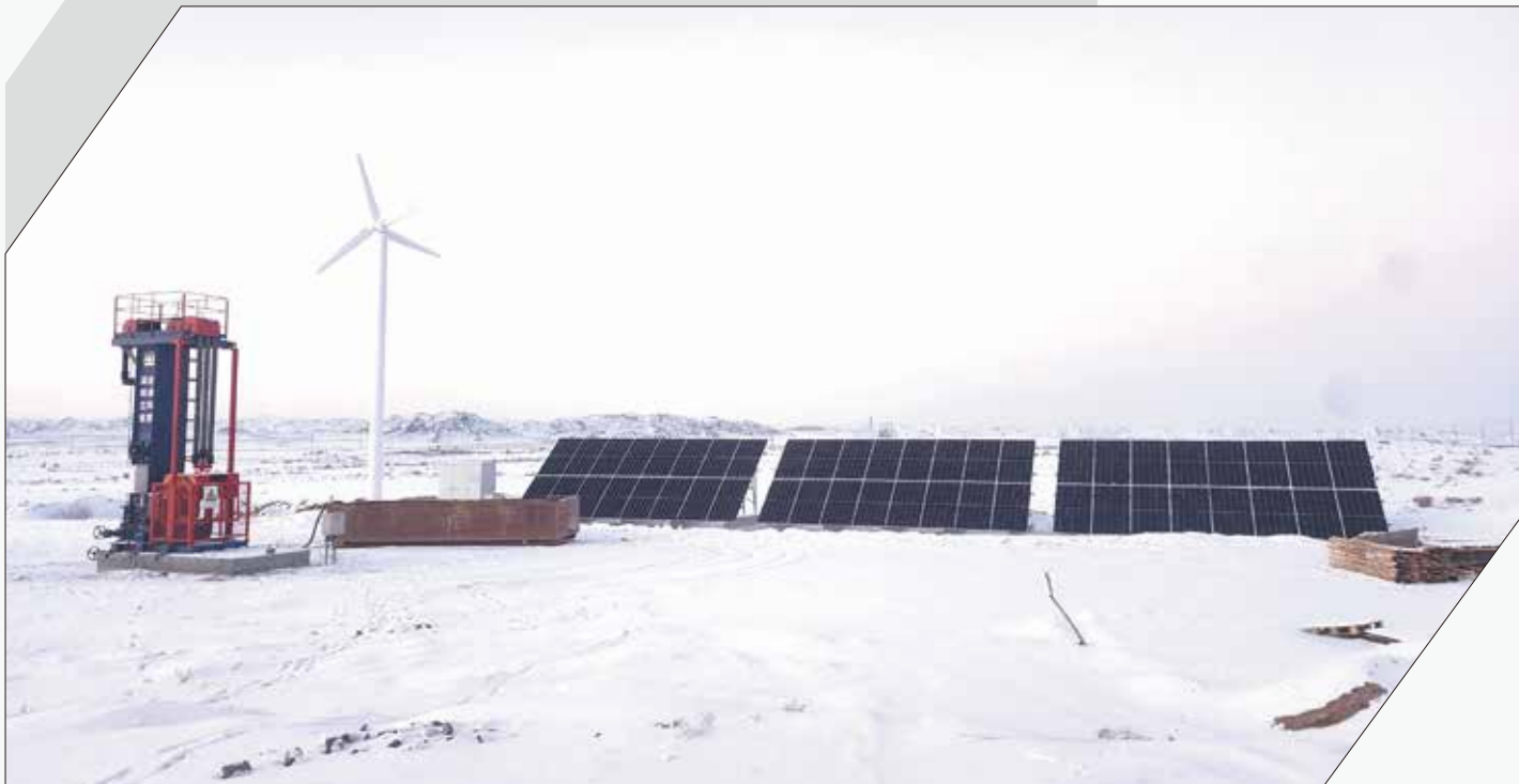
Microgrid System for Oil Extraction in Xinjiang, China
