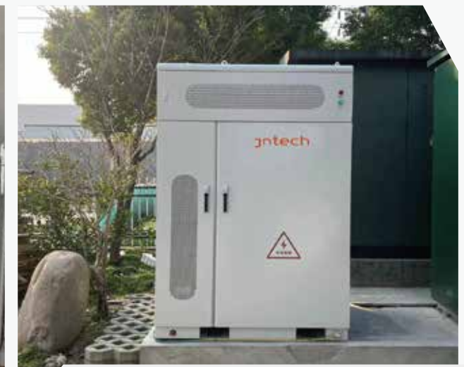
Hefei 100kW/200kWh energy storage system
